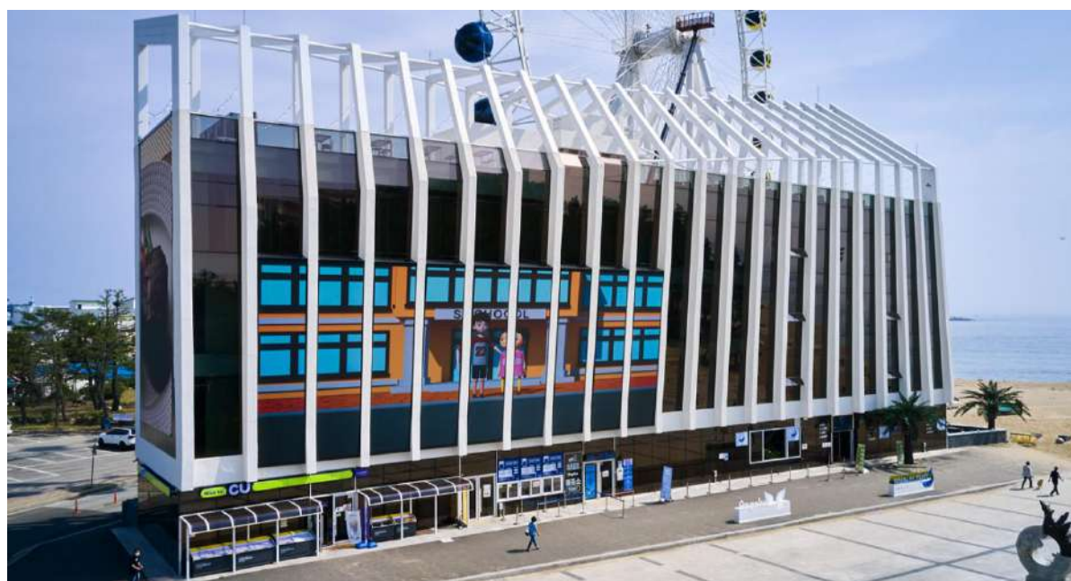
Aluminum screen on the south side of Sokcho coast, Gangwon-do, South Korea (150m 2 )
